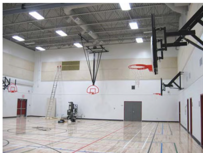
Figure 6. Scissor lift and Tectum panel in Gym B-1.
