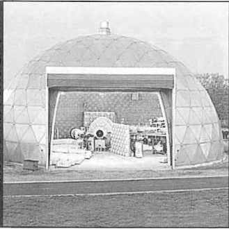
ENGINE TEST FACILITY
