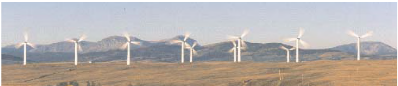
Figure 1. Castle River Wind Farm from the East. Prevailing wind is from the West. (Photo © courtesy of Vision Quest WindElectric ®)
