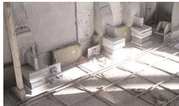
Fig. 3: Pre-Cast Panel Vibration Isolation
