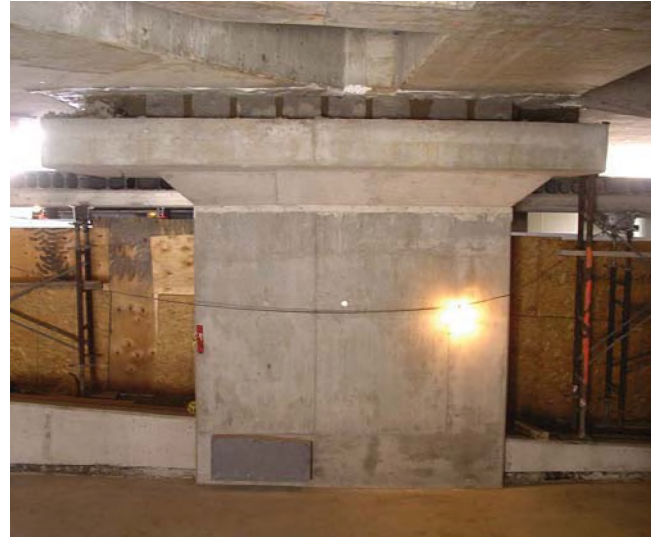
Fig. 2: Column Cap with Isolation Pads; Structural Transfer Grid Visible Above
