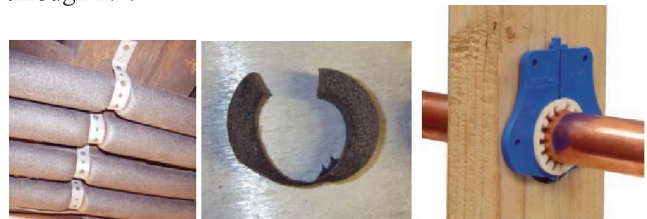
Fig 1.1 Water tubing isolation using foam insulation and successful use of an engineered isolator
