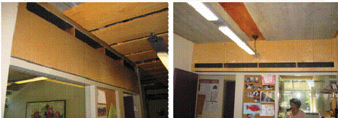
Figure 10: Drawing and photographs of the lined, Z-shaped silencer installed in the Liu office-partition opening.
