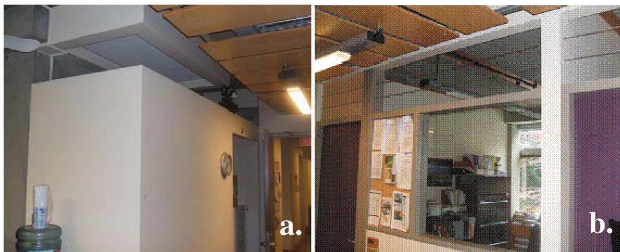
Figure 5: Liu building natural-ventilation system: (a) shafts and floor openings; (b) office/corridor openings.
