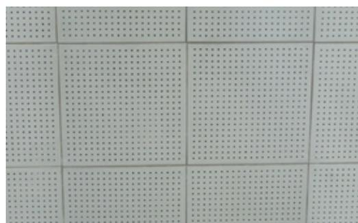
Figure 1: Acoustic ceiling tiles.
