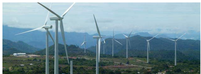
Figure 5. Cerro de Hula, wind power plant in Honduras
