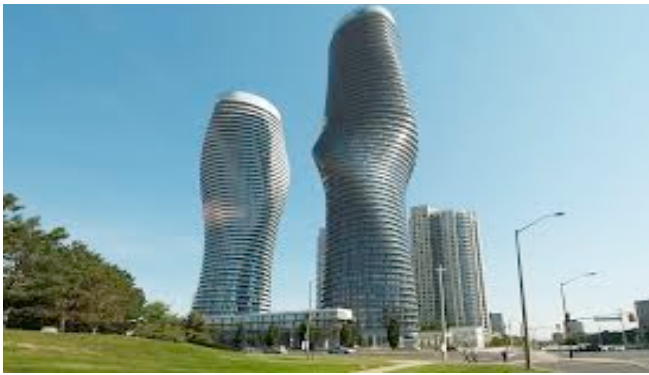
Figure 2. Absolute Towers, Mississauga, Ontario
