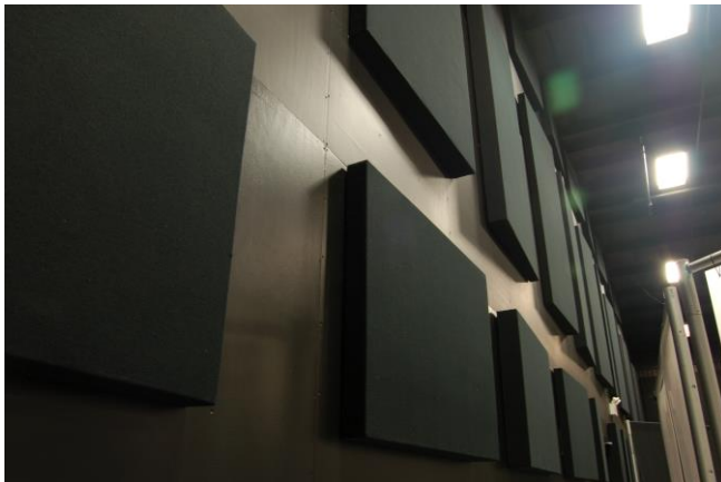
Figure 1: ROXUL insulation is used in Perdue's products; the treatments are then wrapped in fabric or vinyl to meet the acoustic and aesthetic needs of any facility.
