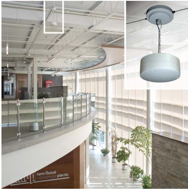
Figure 1: KRM's LogiSon Acoustic Network installed in a facility featuring an open ceiling.
