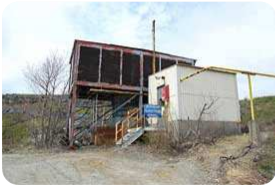
Figure 3: Ventilation system before control
