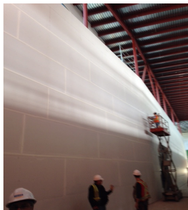
Figure 3: Atrium/Theatre wall under construction - Atrium side.
