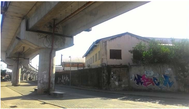
Figure 4: External back view of School #2. Note the proximity to the metro tracks.
