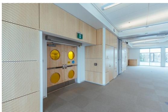
Figure 3: Perforated wood panels backed with duct liner on walls provide additional absorption in multi-purpose room.
