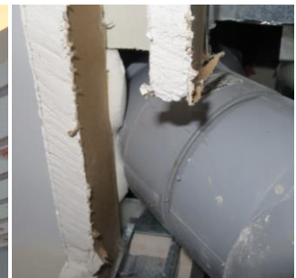
Figure 2: Gypcrete rigidly tying stack to bulkhead
