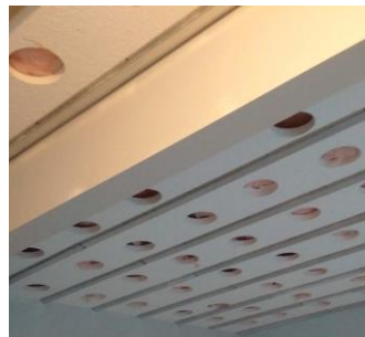
Figure 1: RC channel installed with holes for air
