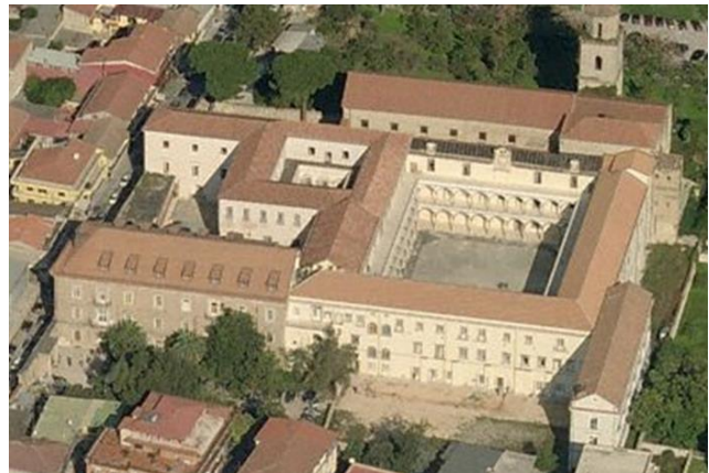
Figure 1: Department of Architecture and Industrial Design aerial view.
