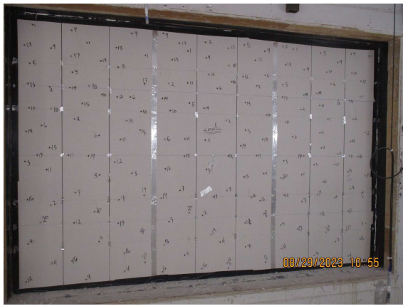
Figure 7: Image of the wall with twenty holes per bay (Case 12), resulting in one hundred and twenty holes in the wall.
