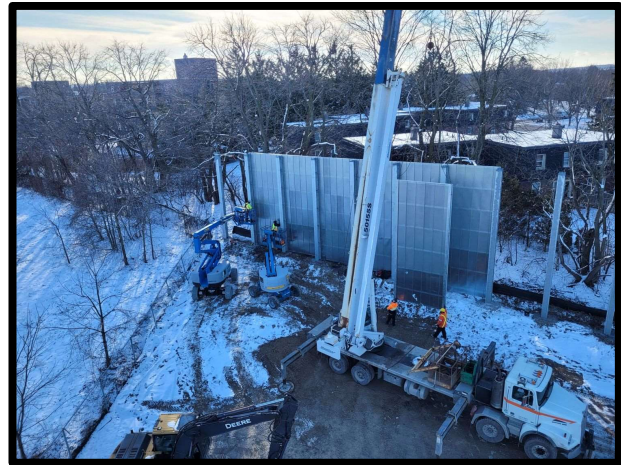
Figure 3: Photograph taken during the install of a large 10 m acoustic barrier.
