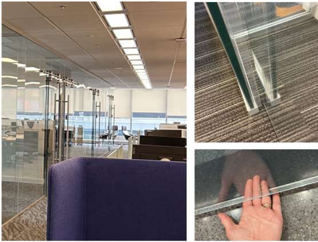
Figure 2: Custom glazed storefront system with typical seals
