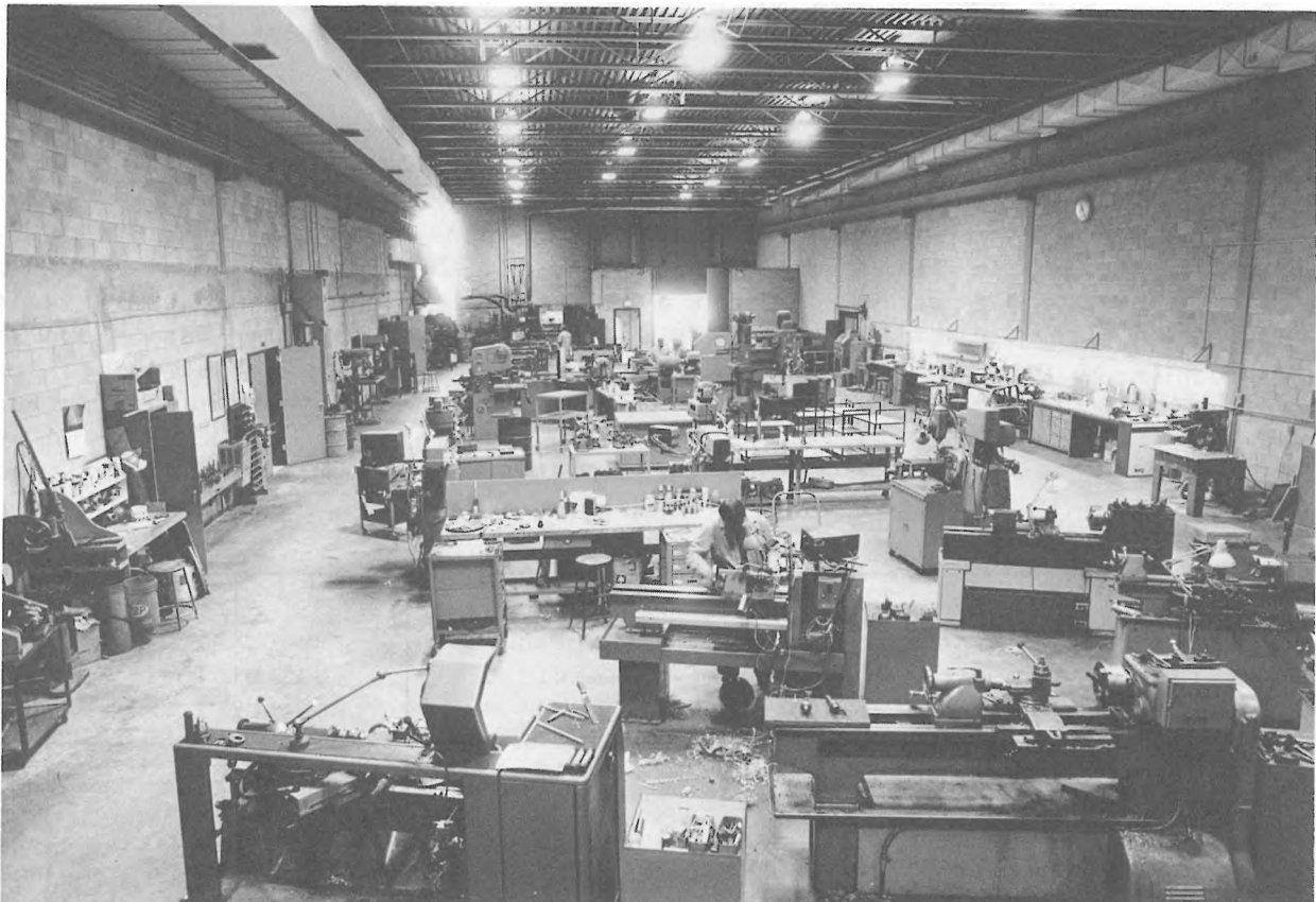
Figure 1 - Photograph of the machine shop showing the room geometry and fitting layout. The partial-height partition is visible at the far end; the doors were closed during all tests.
