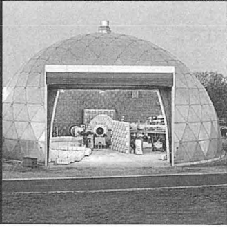
ENGINE TEST FACILITY
