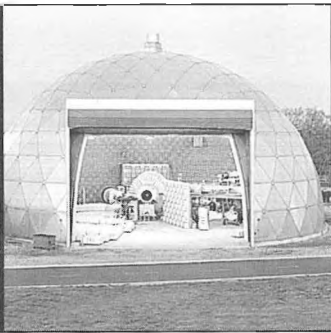
ENGINE TEST FACILITY
