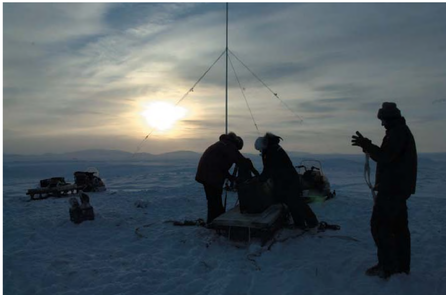
DRDC personnel establish a radio repeater on a hilltop on northern Ellesmere Island
