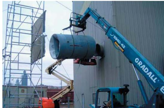
Figure 5. Active Noise Control Silencer
