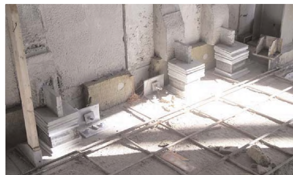
Fig. 3: Pre-Cast Panel Vibration Isolation
