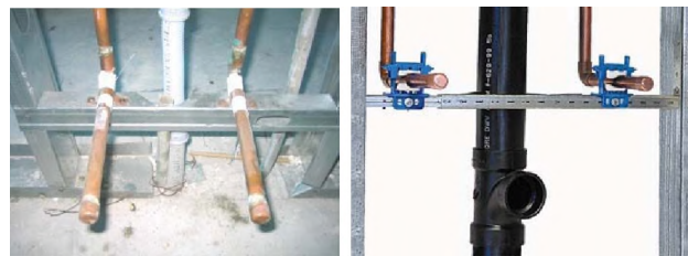
Fig 1.2 Paper compared to an isolated tube clamp
