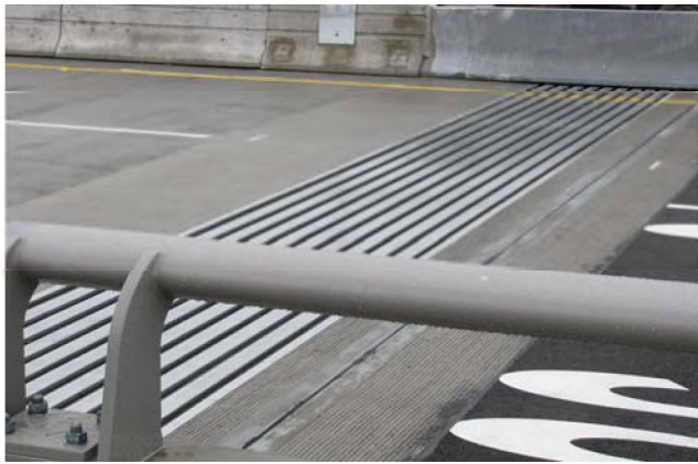
Figure 1. Mageba Modular Expansion Joint
