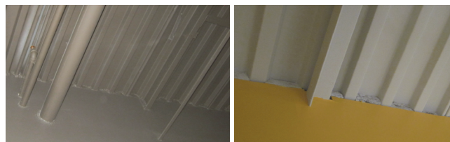
Figure 2: Junction between demising wall and ceiling deck, and penetrations shown sealed (left), and filled but not sealed (right).
