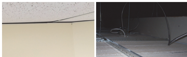
Figure 1: Demising wall shown to extend only to the underside of the ceiling (left), and slightly above the ceiling (right).
