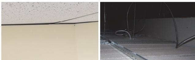
**Figure 1:** Demising wall shown to extend only to the underside of the ceiling (left), and slightly above the ceiling (right).
