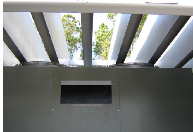
Figure 5: Interior of Enclosure and Pergola Baffles
