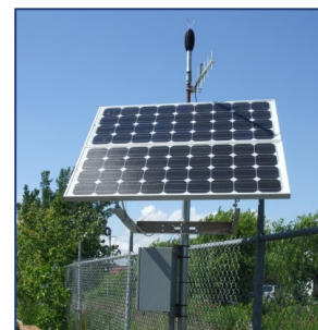
Figure 4: Automated Construction Monitoring System.
