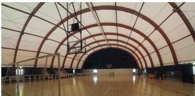
Figure 1: Air dome internal view
