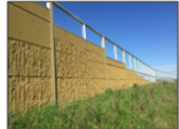
DURISOL PANELS INTEGRATED WITH ACRYLITE SOUNDSTOP
