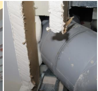
Figure 2: Gypcrete rigidly tying stack to bulkhead
