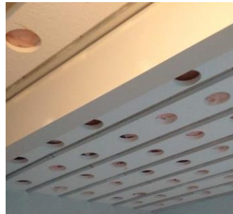
Figure 1: RC channel installed with holes for air
