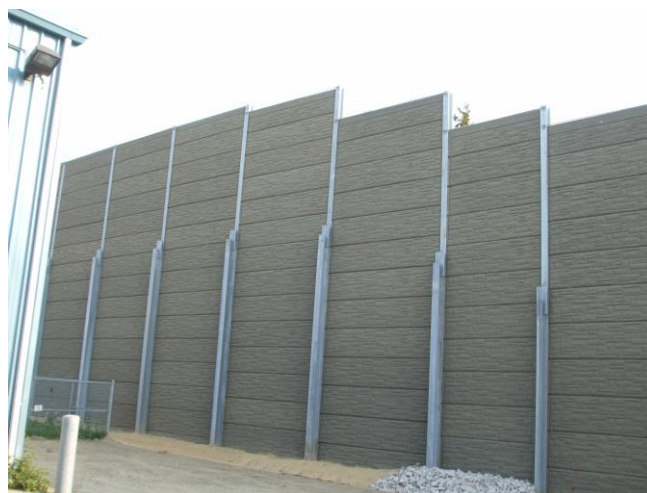
Figure 3: Facility side of noise barrier
