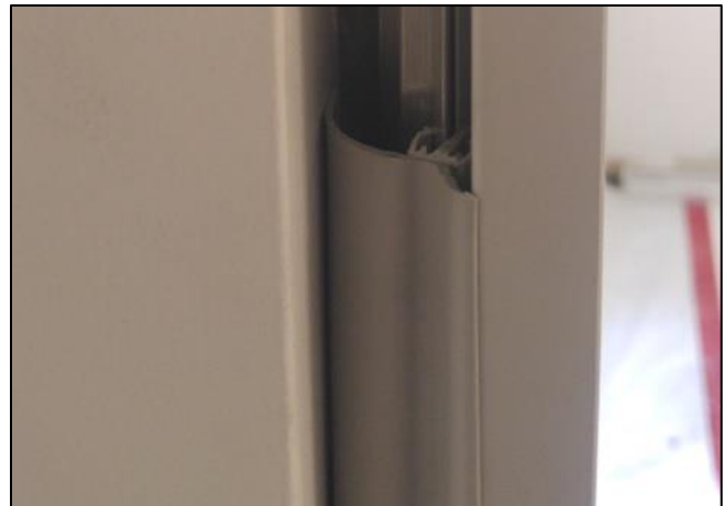
Figure 1: Photograph of PVC “zipper” seal
