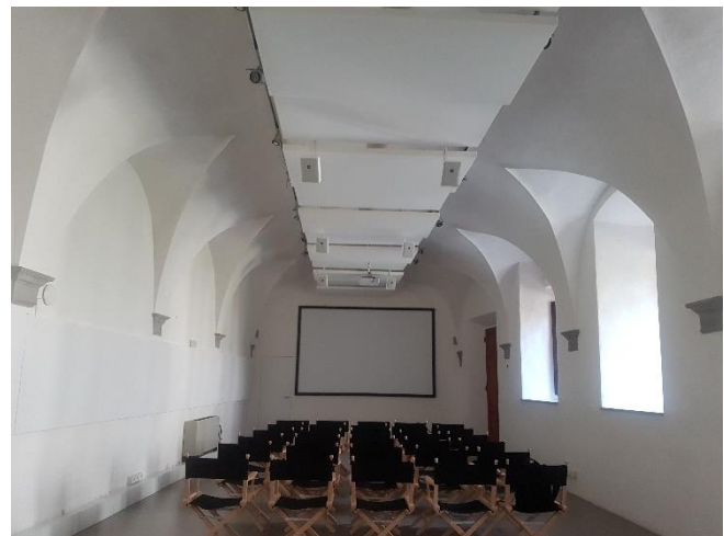
Figure 14: Room in its current state after the installation of the sound-absorbing panels on the side wall and under the vaults.
