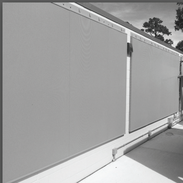
EQUIPMENT YARD NOISE RIGID ABSORPTION PANELS
