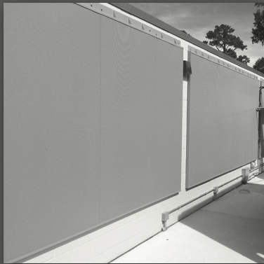
EQUIPMENT YARD NOISE RIGID ABSORPTION PANELS
