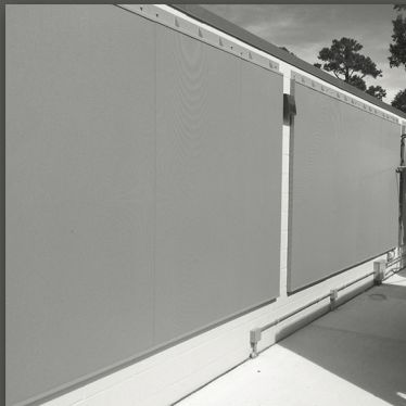
EQUIPMENT YARD NOISE RIGID ABSORPTION PANELS
