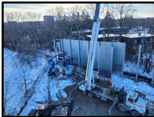
Figure 3: Photograph taken during the install of a large 10 m acoustic barrier.
