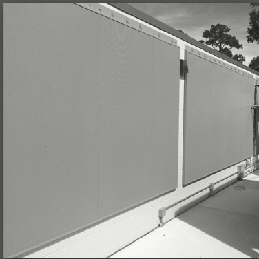
EQUIPMENT YARD NOISE RIGID ABSORPTION PANELS
